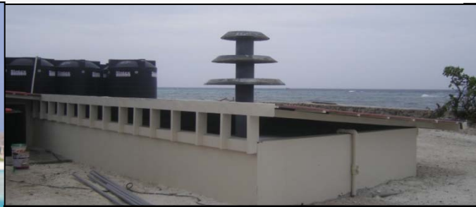
FEED WATER TANK FOR AERATION BEFORE MEMBRANE TREATMENT
