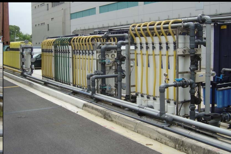
WASTEWATER 10X CONCENTRATION FOR INCINERATION 200 m 3 /day
