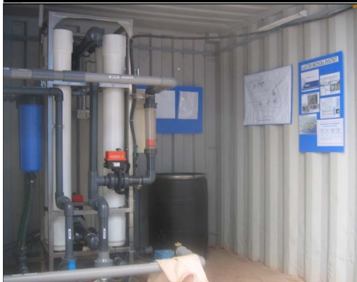
MU-04 SYSTEM (6 m 3 /hr) IN 10FT CONTAINER AT CONDOMINIUM SITE FOR EASY RELOCATION
