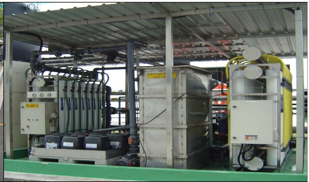
WASTEWATER 10X CONCENTRATION FOR INCINERATION 200 m 3 /day
