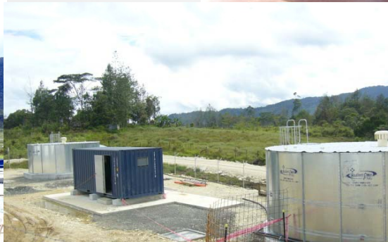
50 m 3 /day MBR-50 High COD Pump Wastewater Treatment Plant
