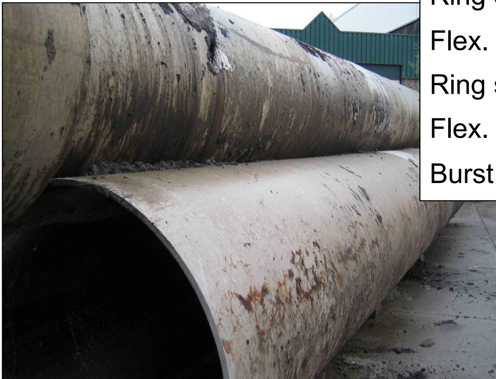
Fig. 1: Two pipes DN 1400 PN 1 SN 5000 excavated after 18 years in operation
